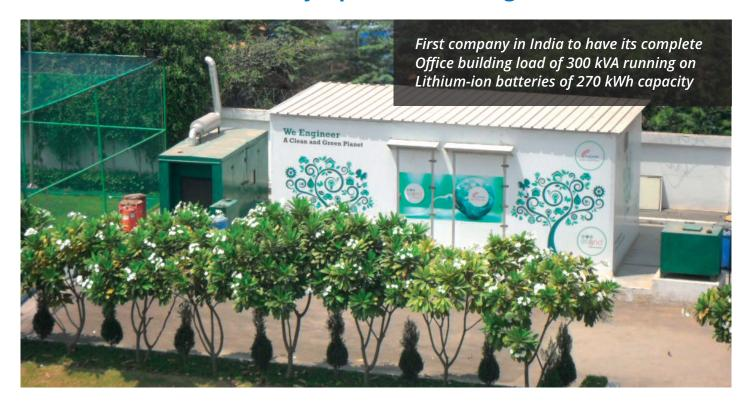
ACME has turned it's headquarter at Gurgaon into one-of-its-kind 'Battery-Operated-Building' in the world through the installation of a technologically advanced energy back-up solution.
