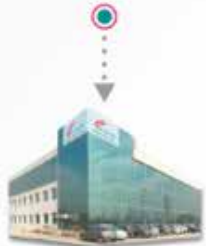
Building on Battery
